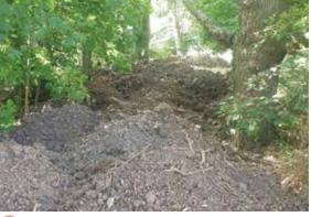
Soil poorly and inappropriately stored within retained tree root zones
