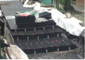
Geotextile and geomembrane run up side of trench
