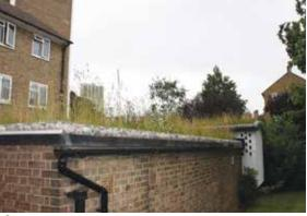
Retrofitted green roof uses existing drainage outlets that were checked for correct sizing
