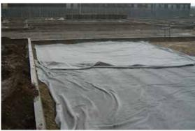
Geotextile - permeable (water will flow through it). Allows water to pass through. Geotextile during heavy rain shows no ponding
