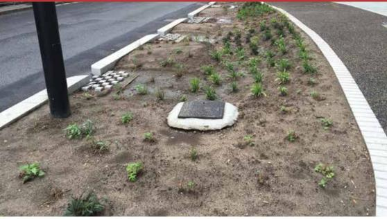
Figure 31.19 Level of soil above the level of inlets from road
