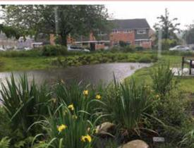
In heavy rainfall, the detention basin has filled up to the level of the outlet, fulfilling its intended capacity
