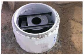
Extra large flow control set at correct levels in a manhole
