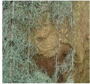
Surface unprepared and matting poorly fitted resulting in erosion behind mat
