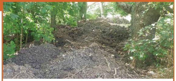
Figure 11.7 Excavated soils being stored within root protection zone of mature trees
