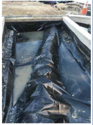
Figure 5.3 Fully-lined SuDS cell used where infiltration could cause migration of contamination. Also note visible existing services running beneath geomembrane
