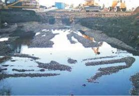
Inadequate formation - poor groundwater control results in difficult excavation and uneven formation
