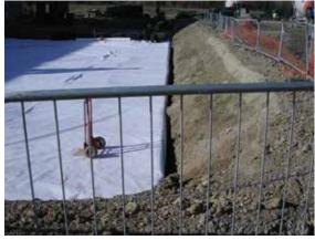
Figure 12.6 Appropriate use of fencing to prevent vehicle access
