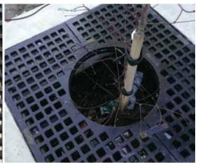
Figure 27.2 Over-filled compacted bioretention planter Figure 27.3
