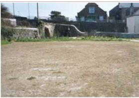
Poor permeability of soil or bedding layer resulting in water ponding on surface and grass dying
