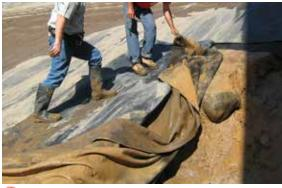
Geomembrane damaged by being laid on top of large projection
