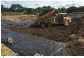
Excavation of SuDS basin in contaminated soils with geotextile separator and clean subsoil being placed
