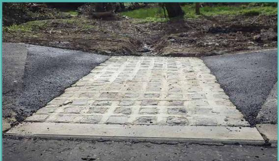
Figure 19.7 Newly re-laid road set at lower level than inlet kerb, restricting surface water runoff from entering the SuDS
