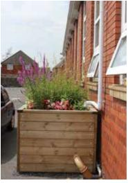
Figure 31.3 Bioretention planter
