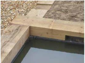
Figure 37.14 Incorrect levels meant water overflowed at Figure 37.15 Levels correct so water flows in right sides instead of to SuDS garden downstream
