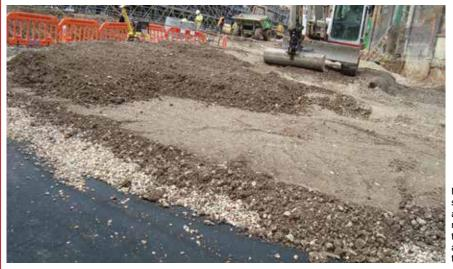
Note the wacker plate seen on thinner layered areas (less than 300 mm), excavator on thicker areas (500 mm+), and the dumper truck off tank completely
