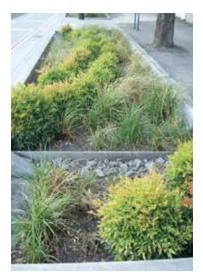
Figure 31.5 Bioretention planter in street
