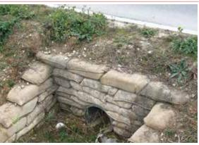
Haunching around kerb does not allow enough topsoil for good vegetation establishment
