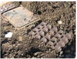
Figure 5.1 Grass reinforced concrete units used on top services lines provide suitable protection
