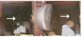
Flow control incorrectly installed on the wrong side of the weir wall. Flow control fitted to the wrong side
