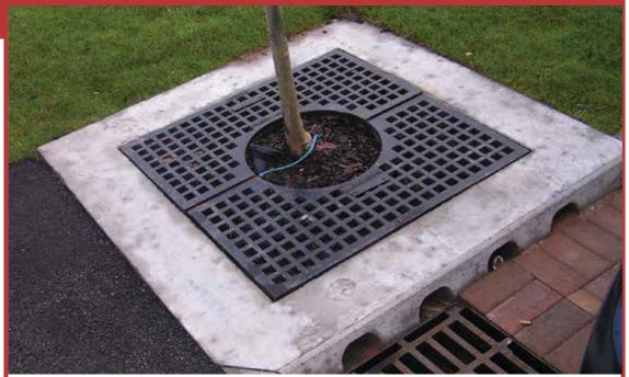
Figure 27.4 Incorrectly positioned bypass inlet
