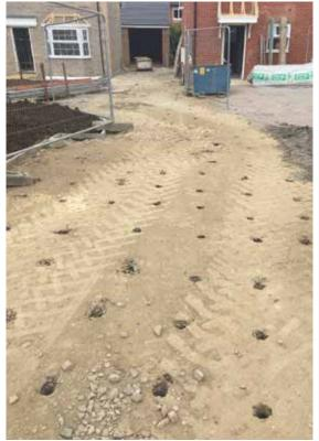
Figure 33.6 Dense bitumen macadam base course not cleaned before coring, and with holes punched in grids, not staggered rows as specified
