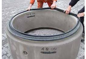
Figure 27.1 Elastomeric seal being correctly stretched into position
