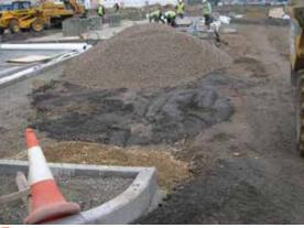
Compaction of subgrade below permeable paving intended to allow water to soak into ground
