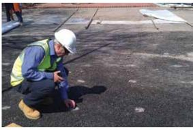
The layer of asphalt is cleaned before coring to prevent mud/site material blocking permeable base, and then filled with granular material to allow drainage, before final permeable finish
