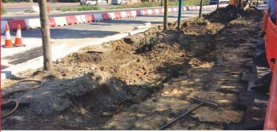
Figure 32.5 Excavation around existing street trees causing root damage
