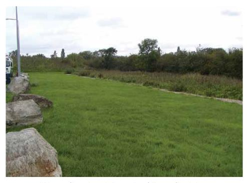
Figure 28.1 Wide grass filter strip on shallow gradient, falling to a filter drain
