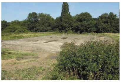
Note that some cells are dry as a result of highly-permeable soil being encountered which was missed during initial soil surveys.
