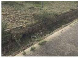
Figure 37.2 Swale formed with coir walls
