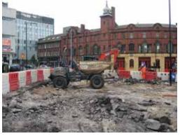
Figure 5.2 Existing asphalt surfaces being broken up
