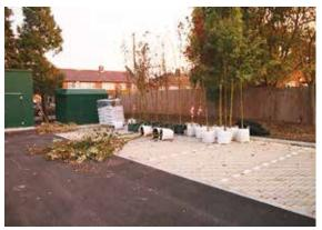
Figure 33.4 Mud and dirt from stored plants can clog pervious surface
