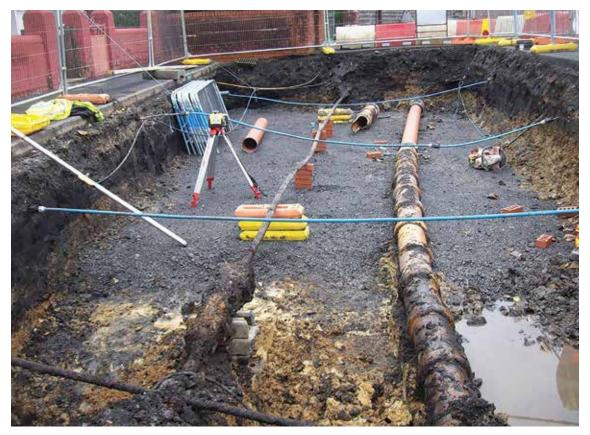
Figure 5.4 Existing underground services can create difficult on-site issues
