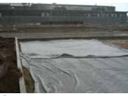
Geotextile – permeable (ie water will flow through it). This allows water to pass through geotextile and during heavy rain shows no ponding
