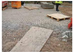
Site materials allowed to spread on finished surface will clog surface and it will need to be remediated
