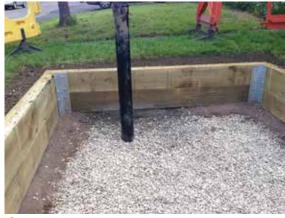
Aggregate laid within bio-retention planter as per specification to allow for good infiltration
