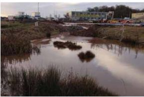
SuDS at end of construction with silt build-up, which had to be removed (and re-graded) before final planting
