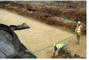
Application of sand and geotextile protection over geomembrane layer
