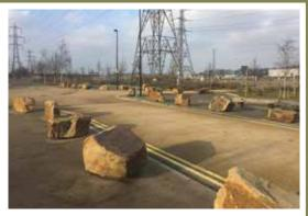
Figure 37.3 Hard channel section within route of swale
