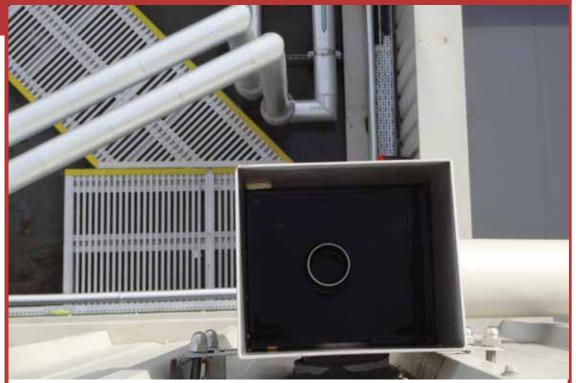
Figure 25.11 Vortex flow control fitted, slowing outlet of water from blue roof and increasing duration of water retention
