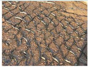
Cellular confinement has not been fully extended before filling
