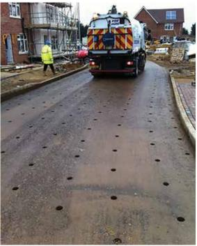
Layer of asphalt used to protect sub-base while it is used for construction traffic then cored before final finishes Sub-base reservoir with contamination of material by fines and soil from nearby bank will clog sub-base
