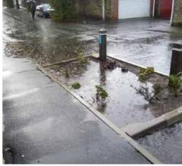
Levels constructed incorrectly and soil not infiltrating through the bioretention system
