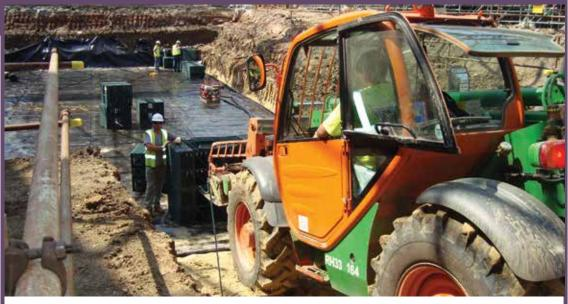
Figure 9.1 Moving attenuation tank units into prepared excavation area
