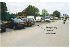
Figure 12.2 Sacrificial sub-base layer allows use of permeable sub-base for parking during construction
