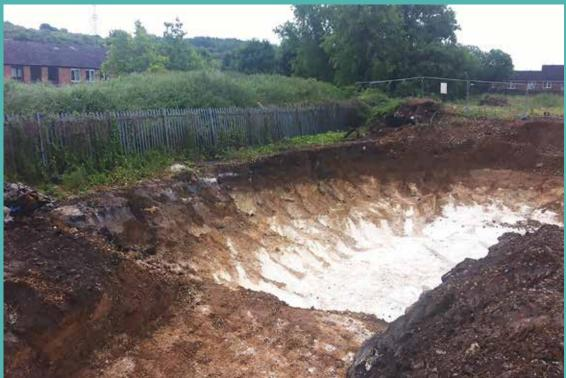
Extensive excavation of polluted chalk before installing the main drainage swale in its place
