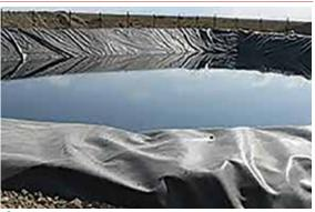
Geomembrane – prevents flow of water (waterproof sheet – normally rubber or plastic)
