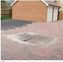
Subsidence of a car park area caused by collapse of attenuation tank
