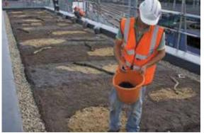
Different substrate materials being placed on a roof to meet biodiversity requirements
