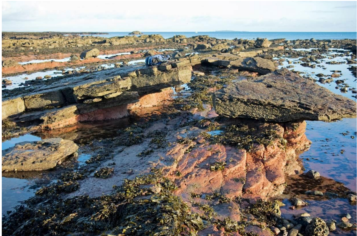
Photo ELC_25 P5: Undercut collapsed blocks on the shore platform south of Great Scar © John Gordon.
