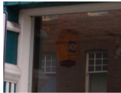
Figure 6 The alarm box on this cafe is positioned on the wall behind the fanlight reducing its visual impact on the exterior of the building while still acting as a deterrent
