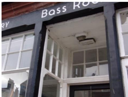
Figure 5 Positioning the alarm behind the light in the ceiling of the shop doorway reduces its visual impact while still acting as a deterrent
