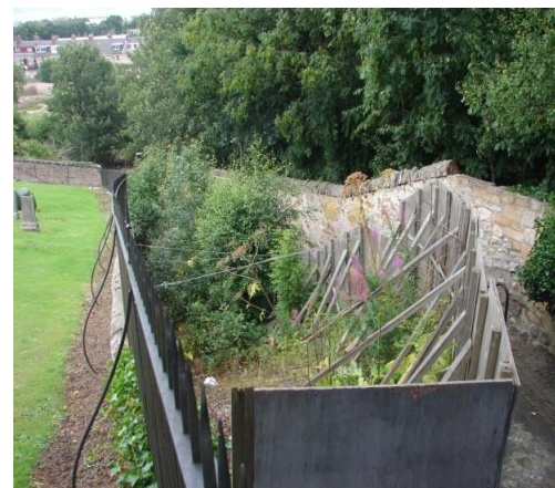
Figure 101 The walls at the graveyard on the edge of the brae have been hoarded off for many years and require repair
