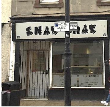
55 High St: Before improvement
