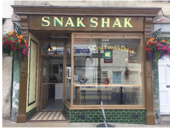
55 High St: After restoration with a signwritten sign. The owner reported an increase in business after work was done.
