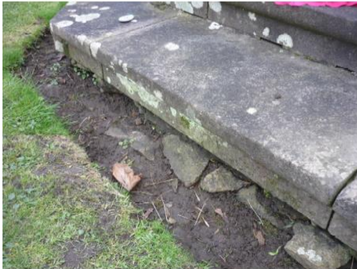
War Memorial suffering from erosion and requires repointing
