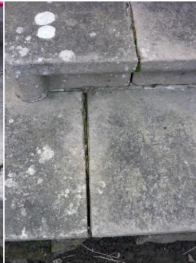
War Memorial suffering from erosion and requires repointing
