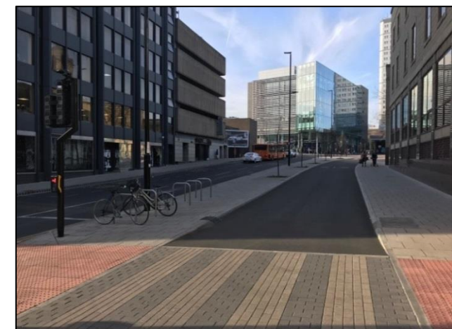
Figure 2-17: Dual Carriageway Converted to Single Carriageway with Cycleway, Newcastle
