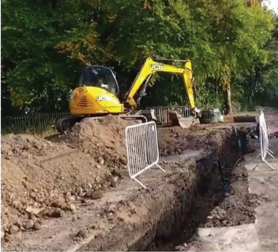
Installation of pipes for ground source heat pump at Saughton Park. Image credit: Pete McDougall / City of Edinburgh Council
