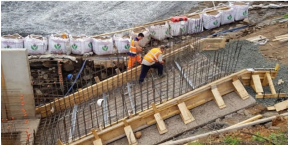
Installation of dam for micro-hydro at Saughton Park. Image credit: Pete McDougall / City of Edinburgh Council
