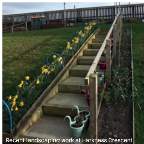
Recent landscaping work at Harkness Crescent
