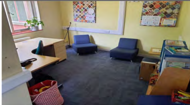
Photo 9: Concealed bitumen-based flooring adhesive (Chrysotile): Sample No: S0055: Room No: B01/FG/R009: Auxiliary Room
