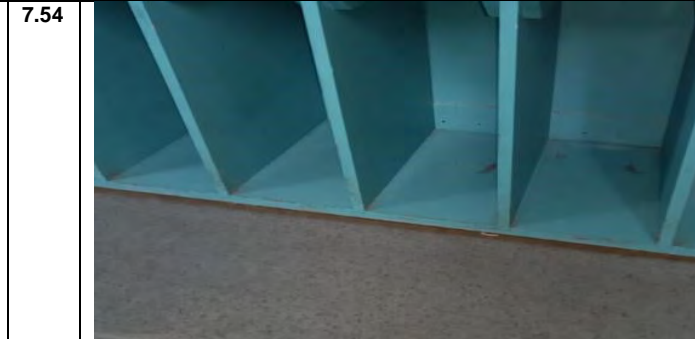
Photo 54: Concealed asbestos skirting boards (Chrysotile): Sample No: S007: Room No: B01/F1/R022: Circulation Area
