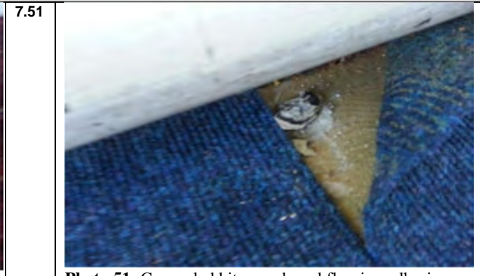
Photo 51: Concealed bitumen-based flooring adhesive (Chrysotile): Sample No: S004: Room No: B01/F1/R013: Classroom
