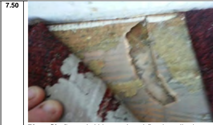
Photo 50: Concealed bitumen-based flooring adhesive (Chrysotile): Sample No: S003: Room No: B01/F1/R012: Classroom
