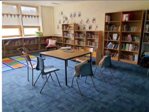
Photo 14: Concealed bitumen-based flooring adhesive (Chrysotile): Sample No: S010: Room No: B01/FG/R025: Library
