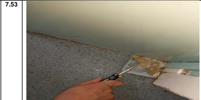
Photo 53: Concealed bitumen-based flooring adhesive (Chrysotile): Sample No: S008: Room No: B01/F1/R022: Circulation Area
