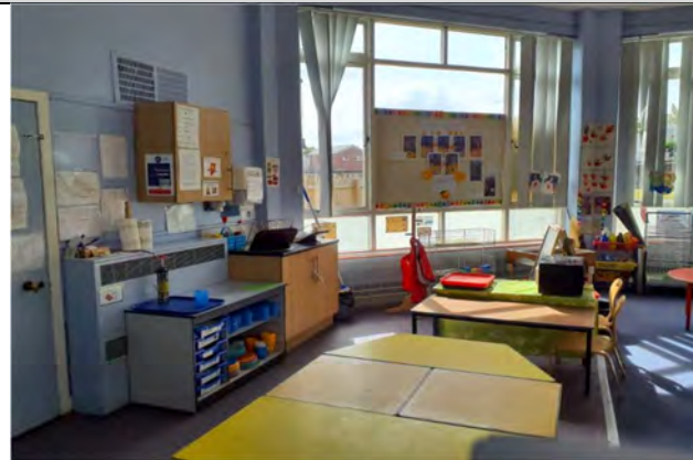
Photo 8: Concealed red floor tiles below fan convactor radiator (Chrysotile): Sample No S0048: Room No: B01/FG/R008: Classroom
