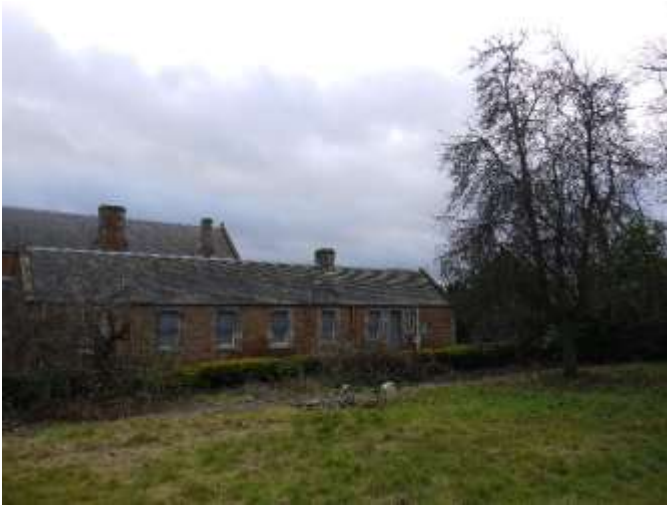
Ancillary Building north elevation
