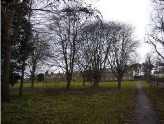
Main building and pavilions' south elevation, viewed from footpath on the east of the Site
