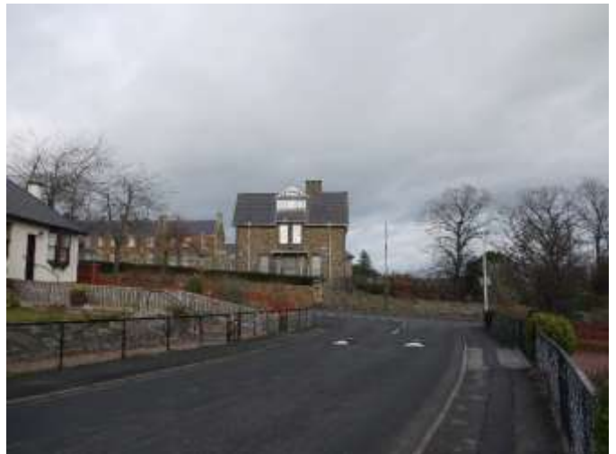
Main building and south-west pavilion from Davidson Terrace
