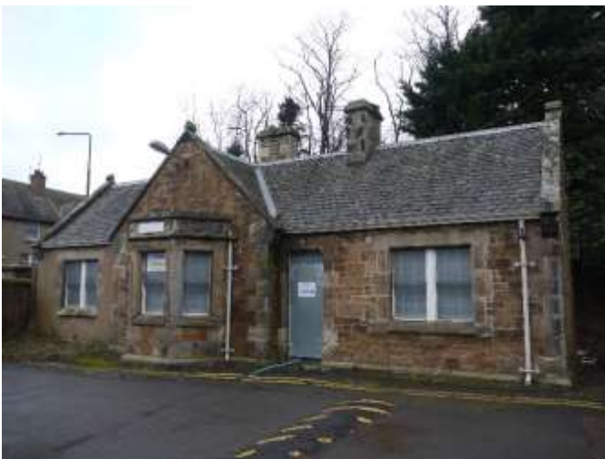
North Lodge, south elevation
