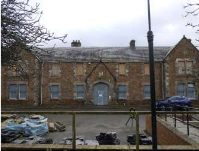
North, entrance elevation
