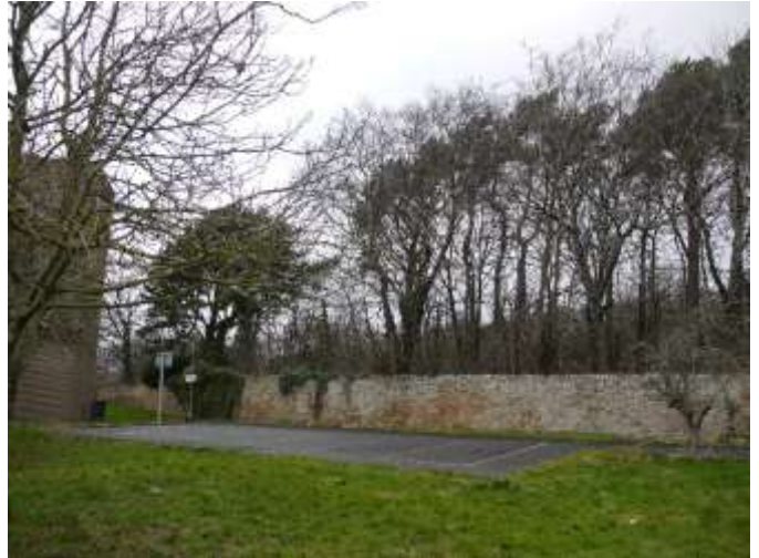
Northern boundary wall
