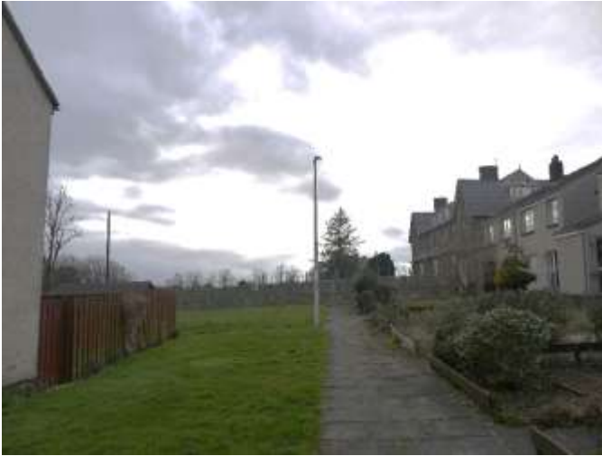
South-east pavilion and grounds viewed from Herdmanflat
