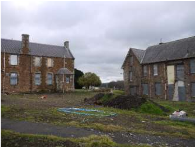
Area west of main building, north of south-west pavilion (with former modern infill demolished)
