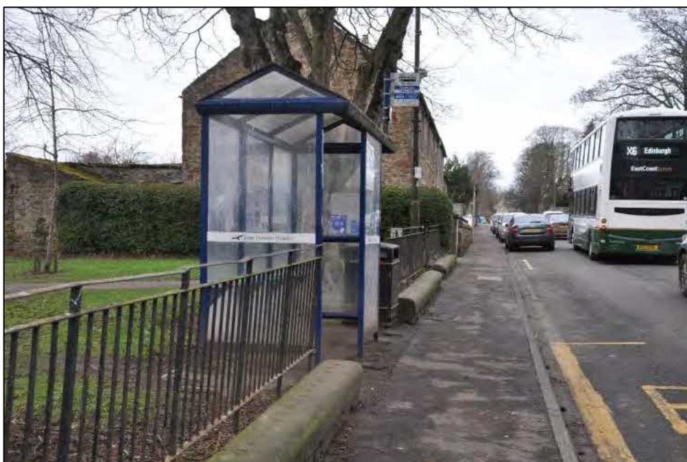
Figure 3-8 : Station Road Westbound Bus Stop
