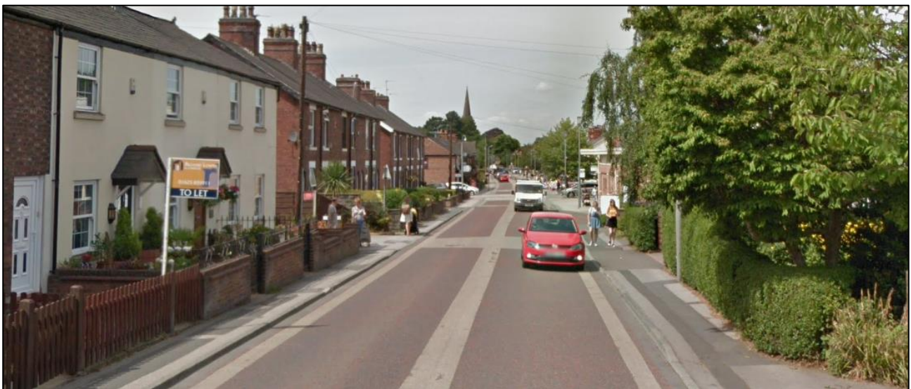
Figure 2: Example mixed traffic street treatment with narrowed lanes
