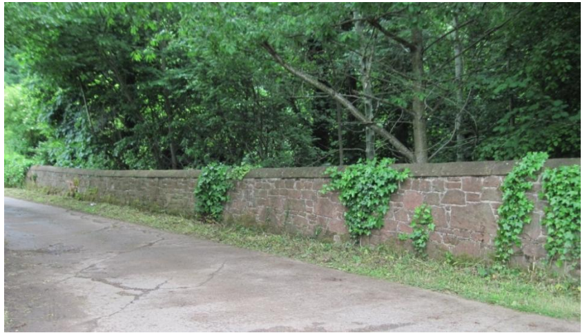
Typical red sandstone wall to bridge
