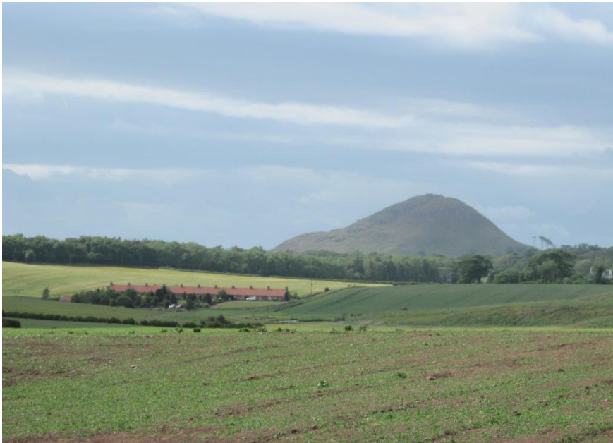
Listed buildings of Redside Farm Cottages, single-storey, stone-built, pan-tile roofs set within rolling fields between crags and influenced by North Berwick Law
