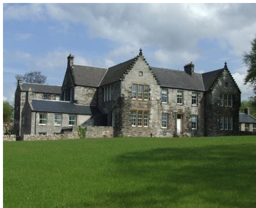
Figure 58 Wedderburn House dates from 1861 and was converted to apartments, 2002
