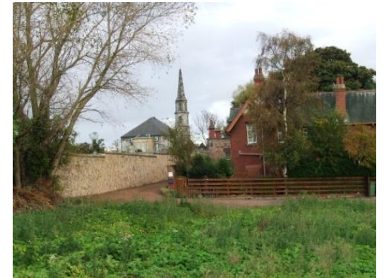
Figure 45 The house on the right was originally one of the service buildings for St Michael's House and like the main house is constructed of red brick. The graveyard wall adjacent was recently repaired.
