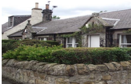
Figure 102 The right hand cottage of this pair on Crookston Road is missing its decorative stone porch finial
