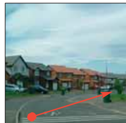
Example illustrates that bend and horizontal carriageway displacement is not combined with a vertical measure to obscure the long sightline. The driver still has long sightline, encouraging higher vehicle speed.
