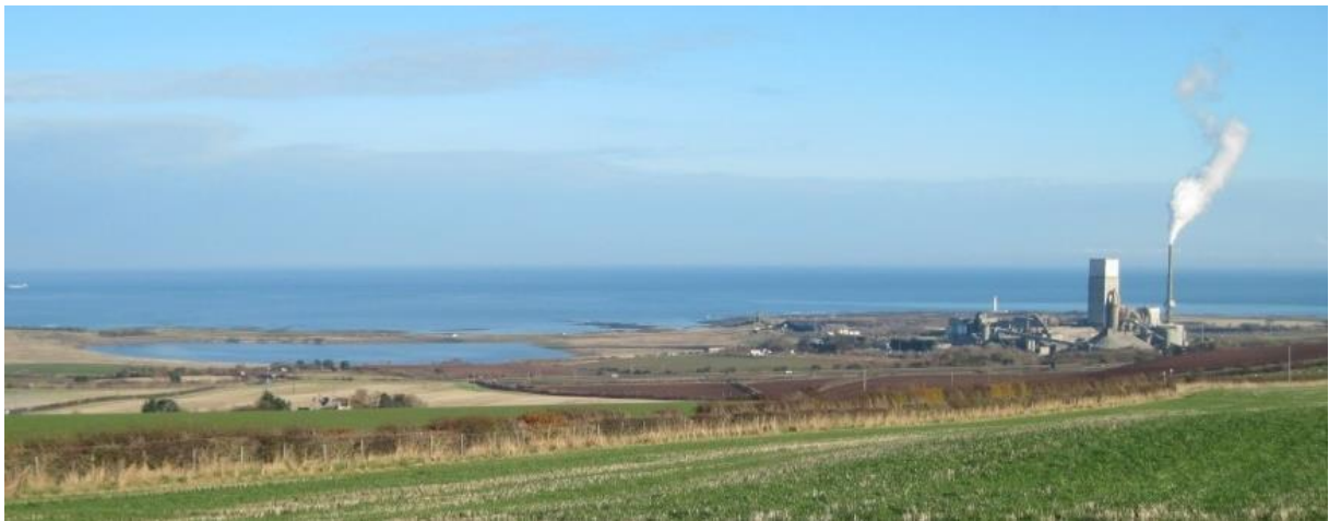
Cement works and infilled quarry in its low lying coastal setting
