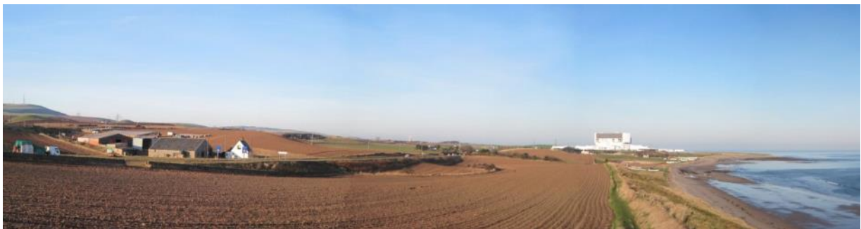
Torness Power Station set within the arable landscape and coast with the plain rising towards the hills to the west
