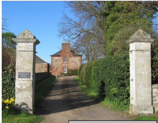
Morham Bank Farmhouse
