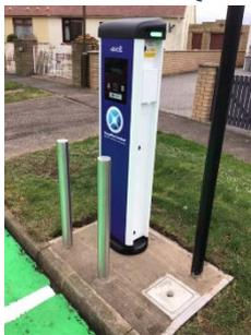
These 22.5kW chargepoints usually have two sockets on a single unit. They are installed between 2 parking bays so that 2 vehicles can charge at once. They tend to be fairly unobtrusive compact units. Where a Destination chargepoint is referred to in this document this will be a double-outlet unit with two designated parking bays.
