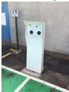
These (7.4kW) units take 6-8 hours to fully charge a vehicle, and are therefore less suitable for areas where high turnover is required and the parking time is restricted. However, they are useful for workplaces and long-stay car parks. In 2018, ELC replaced all of our dated Standard public chargepoints with Destination (Fast) or Journey (Rapid) chargepoints. ScotRail, and other private hosts still install new and operate existing Standard chargepoints.
