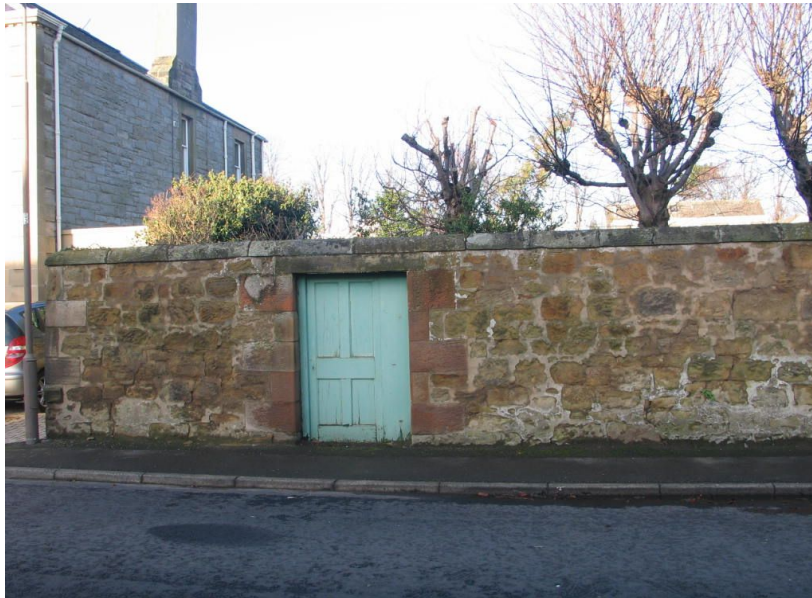
old gate in wall now redundant
