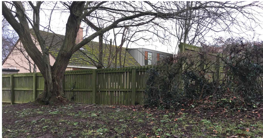
Winter view 01 of rear of 13 & 14 Roodwell Cottages from footpath to the West showing proposed roof alteration.
