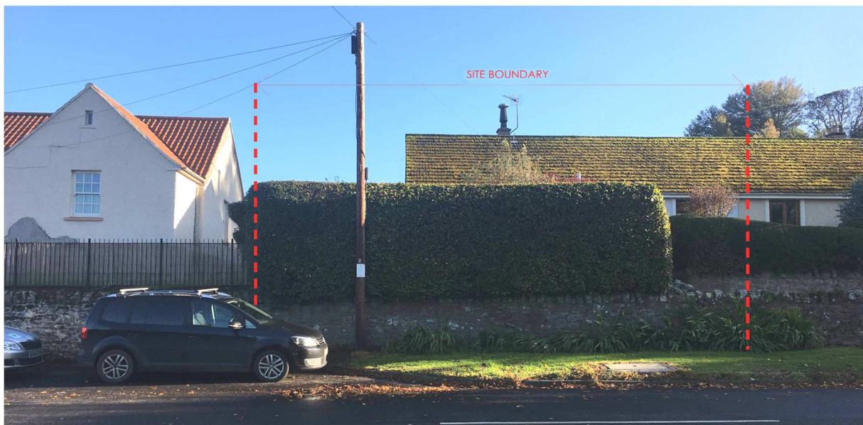
Front of 13 Roodwell Cottages view.
