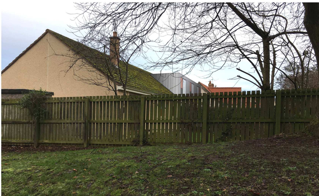
Winter view 02 of rear of 13 & 14 Roodwell Cottages from footpath to the West showing proposed roof alteration.
