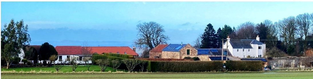
Clearly part of the cluster of homes at West Garleton, Nouster Cottage (left) is neither isolated nor sporadic.
