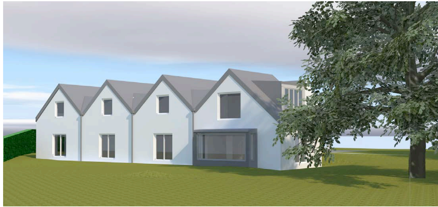
View of new four gabled extension to North
