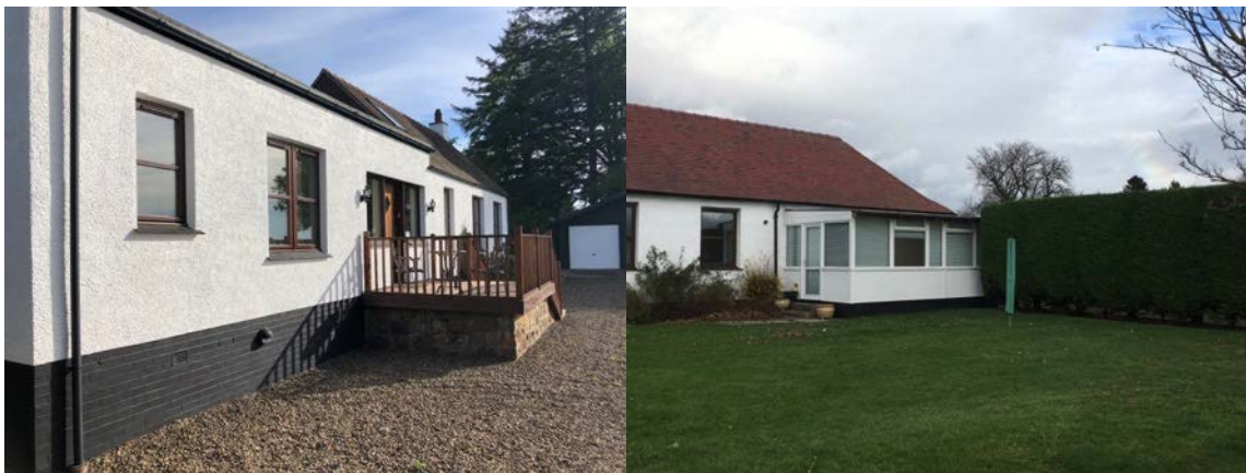
Flat roof extension and conservatory added to the original cottage
