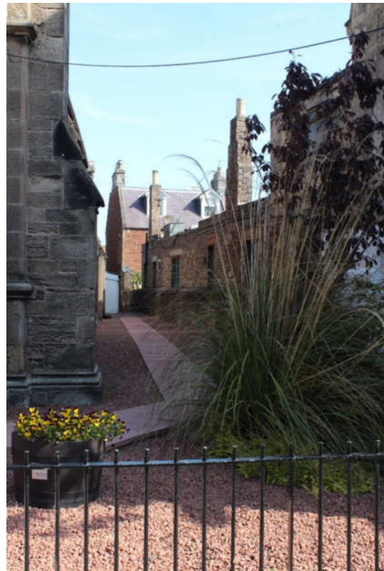
4. 59 Forth Street viewed from High Street
