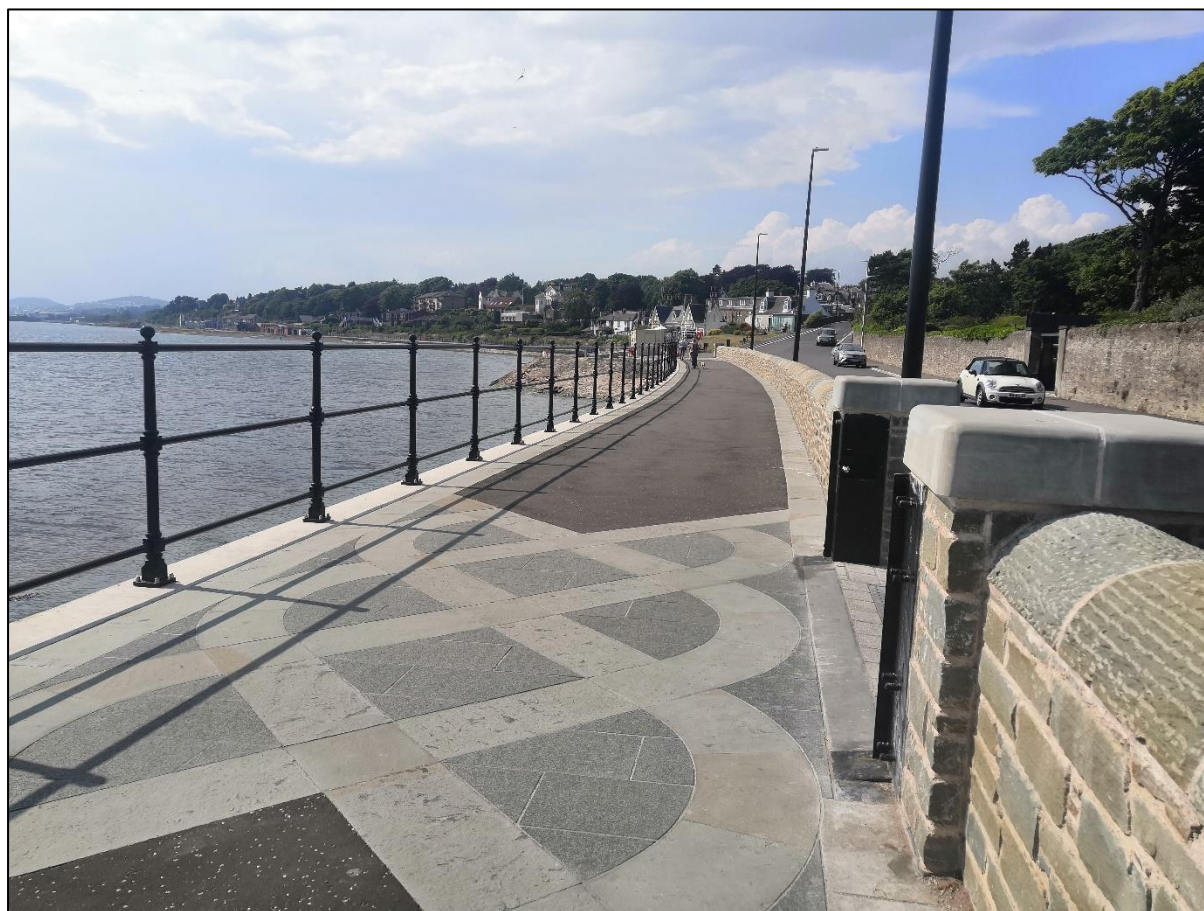
Figure 2.2: Active travel facility adjacent to new flood wall, Broughty Ferry
