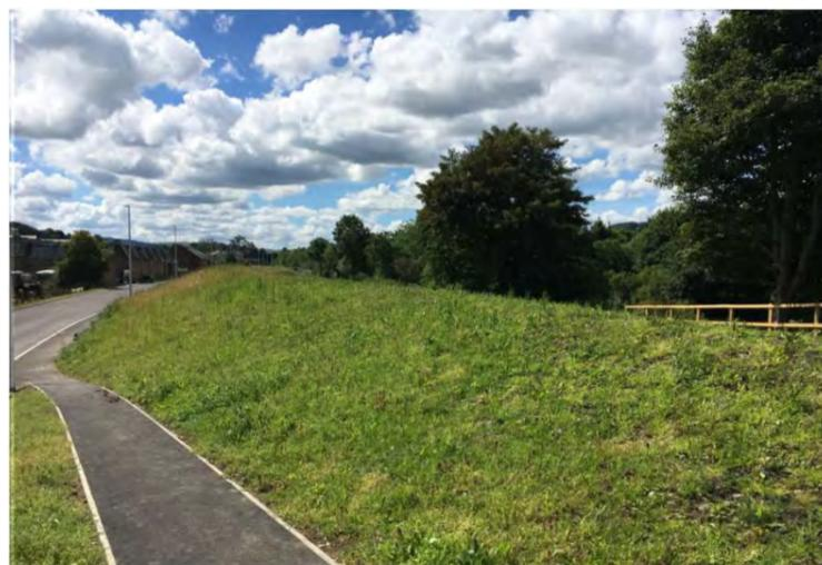
Example of a ramped path over a flood defence embankment
