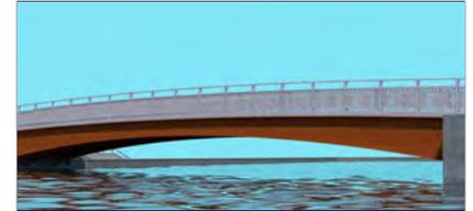
Example of a composite timber-steel multi girder footbridge
