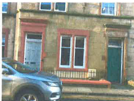
■ Balfour Street, North
