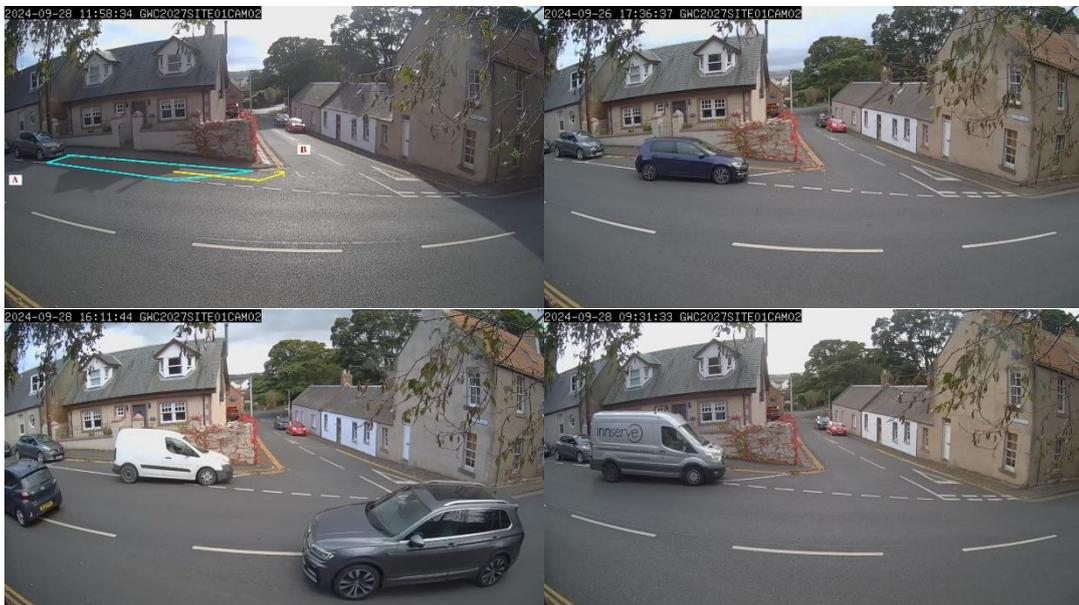
Figure 8-1: Examples of vehicles overrunning the corner at Brewery Lane
