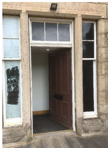
Images of the current property (from left to right), The rear bay window unsympathetically altered, Front door where the openings are decaying, Inside the main Banking Hall showing no architectural merit.
