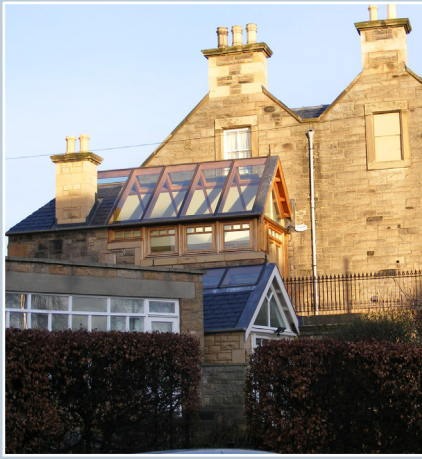
An extension to a house in a conservation area, set back from the front elevation, of glass and timber that echoes conservatories in the area.
