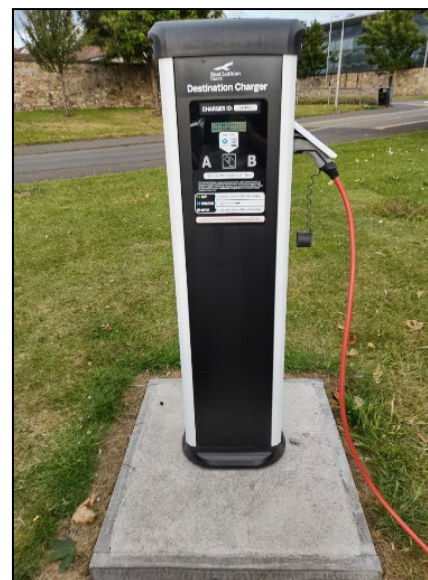
Figure 5.2 - 7-22kW Destination Charger
