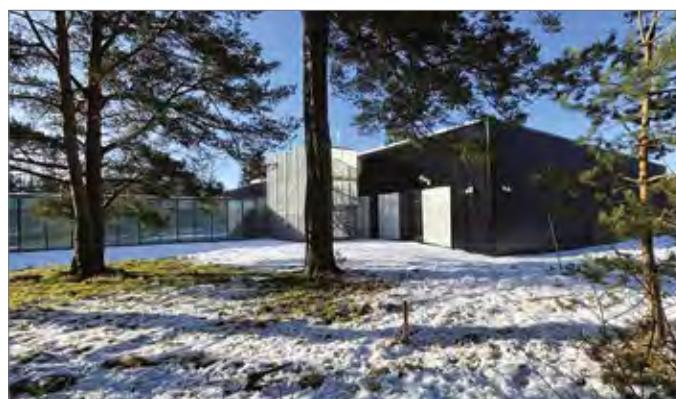
Edinburgh International Data Facility
