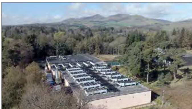
Advanced Computing Facility from the air
