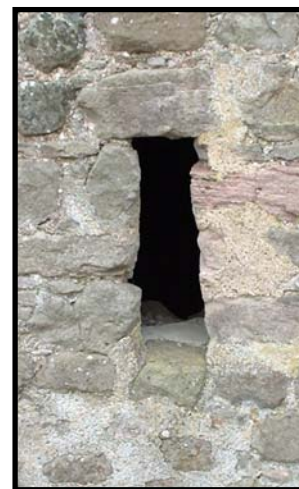
Ventilation slot, Bankhead, Humberie
