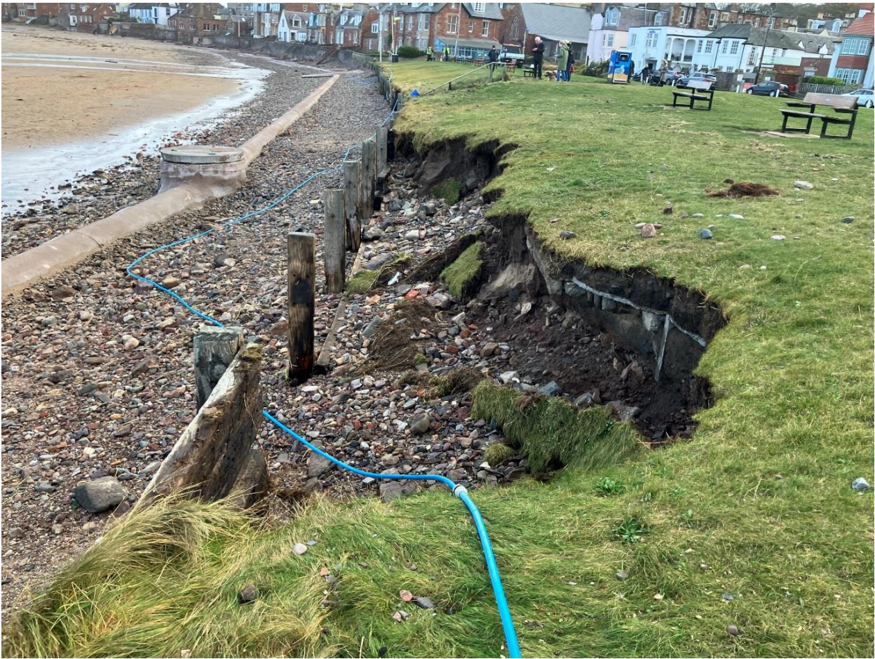
Coastal erosion affecting West Bay Beach, North Berwick
