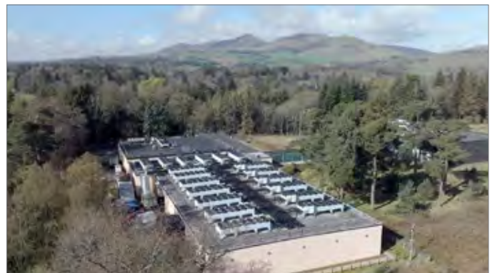
Advanced Computing Facility from the air
