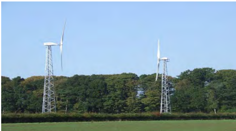
Lattice Tower and Twin Bladed Turbine
