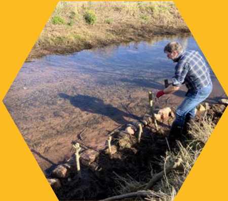
Path Wardens at Thorntonloch repairing the willow banking.
